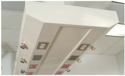
Overhead Service Enclosures
